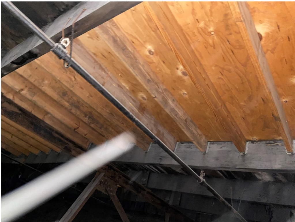
AREA W/ NEW DECK REPAIRS TO BE REPLICATED
