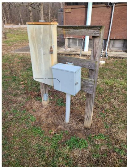
LOWER LOOP AREA NORTH SIDE ELECTRICAL RACK - REPLACE OUTLET WITH PERMANENTLY MOUNTED WEATHERPROOF OUTLET
